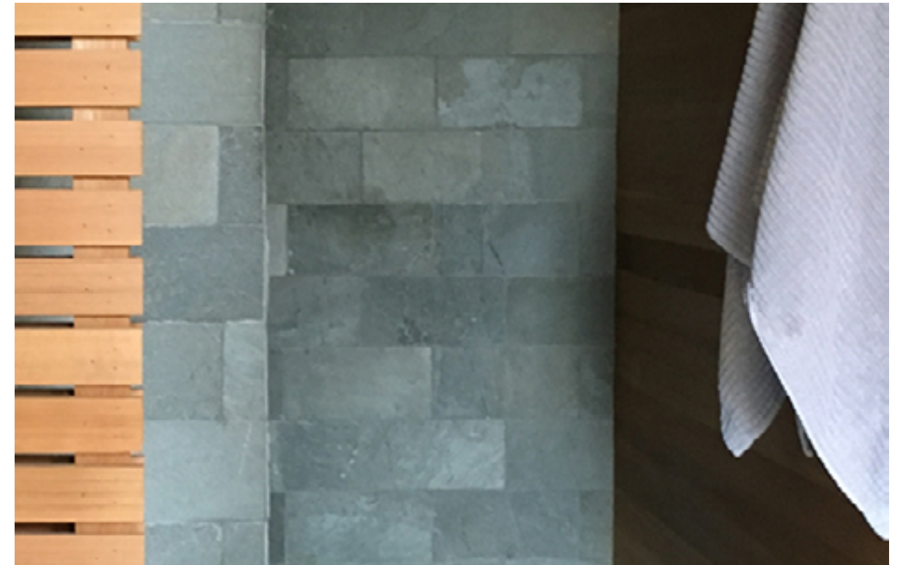
Pictured above is the grey quartzite tile, installed from floor to ceiling in the master bathroom shower.
