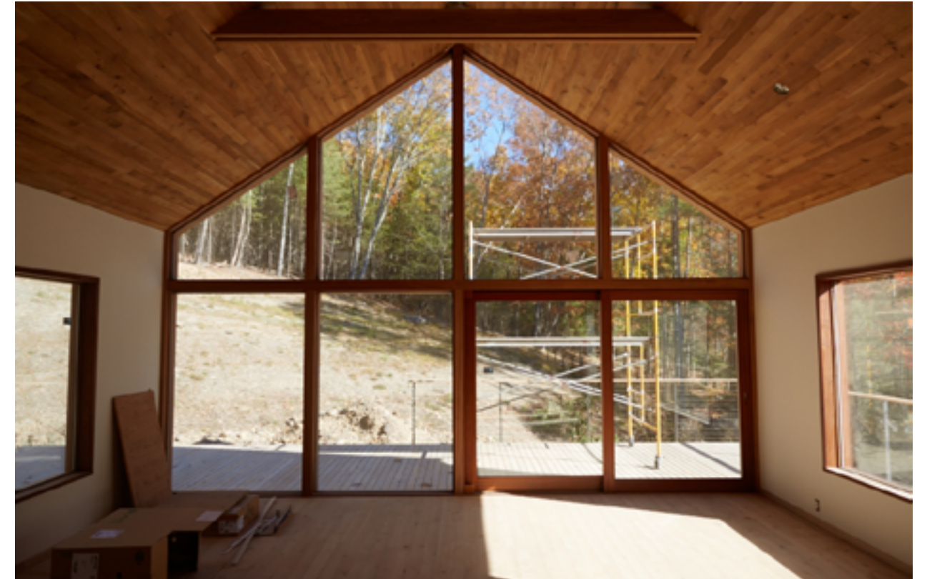
Near completion, the uninterrupted window wall in the great room of the model house at Hudson Woods.
